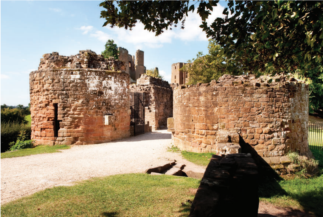
A recent photograph of the remains of Mortimer's Tower, the main gatehouse to Kenilworth Castle, which was built in King John's reign.
