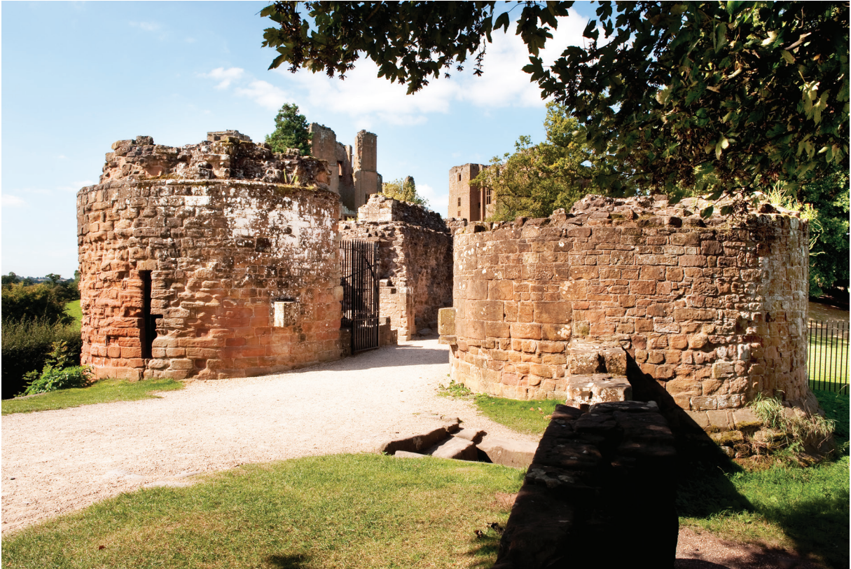
A recent photograph of the remains of Mortimer's Tower, the main gatehouse to Kenilworth Castle, which was built in King John's reign.
