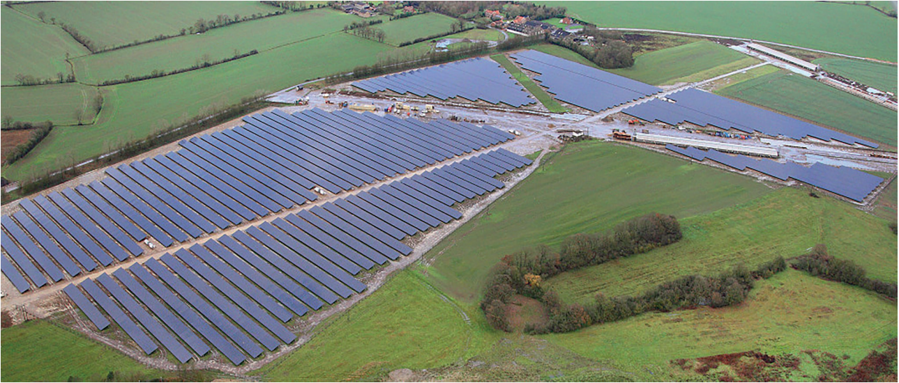
Fig. 3a – A solar farm near Ipswich
